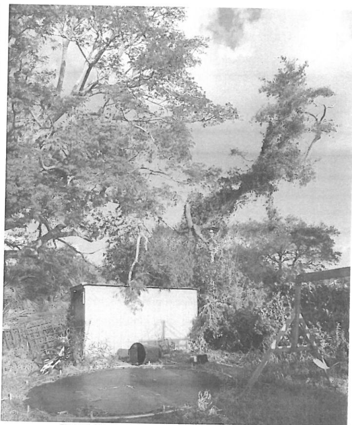
Figure 4 701 W. Winifred with Irma damage to shed and fence
